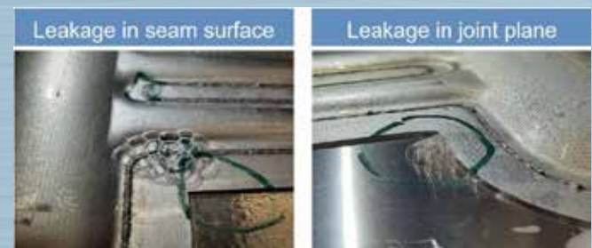
Figure 9: Different types of leakage in cooling plates welded with the standard process.
